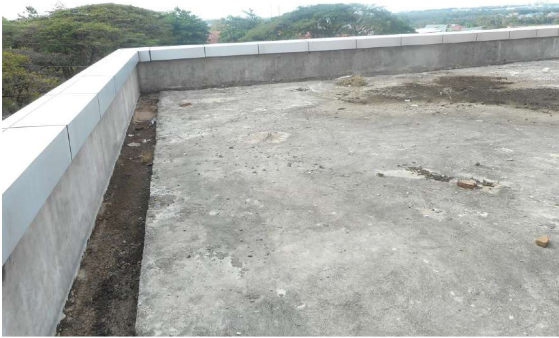
Photo 11 - Story 5 Podium Concrete Roof and Drainage
