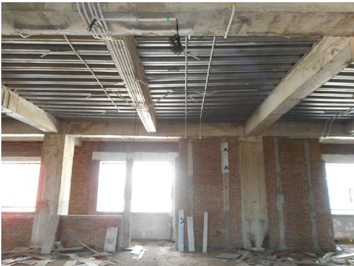
Photo 6 - Story 3 Deformed beam
