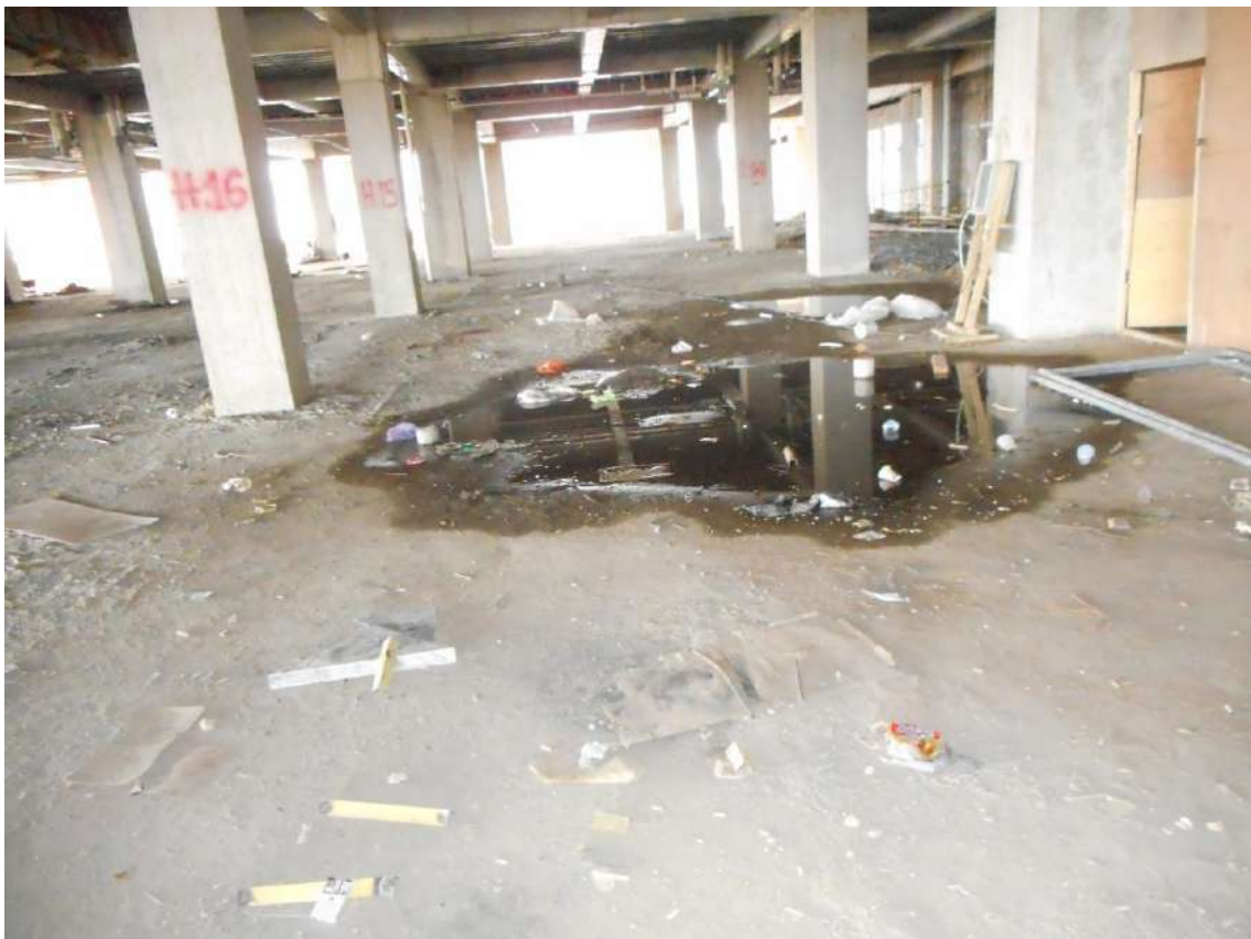
Photo 4 - Story 2 Ponding Water
