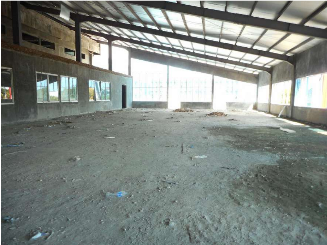
Photo 7 - Story 3 Podium Steel Roof
