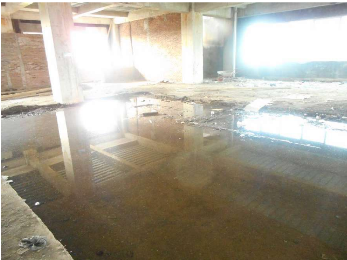
Photo 10 - Story 5 Ponding Water
