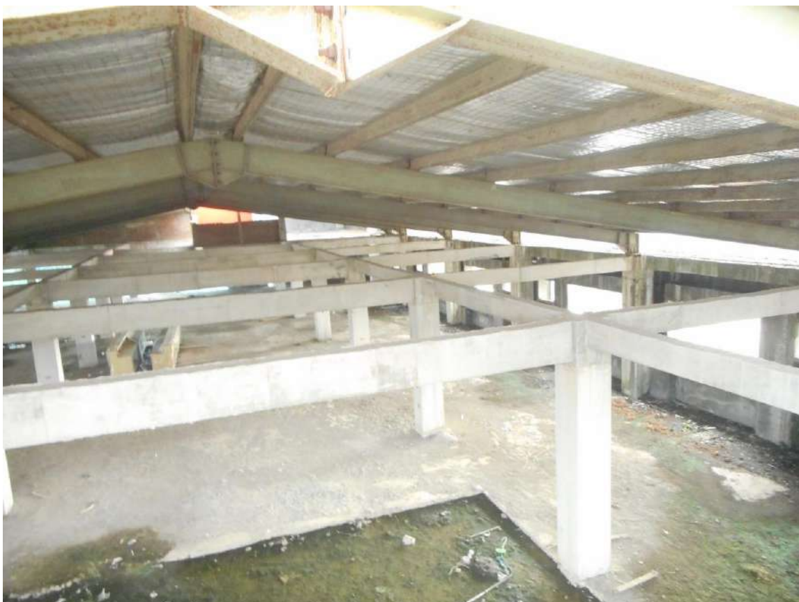
Photo 12 - Story 6 and Steel Roof
