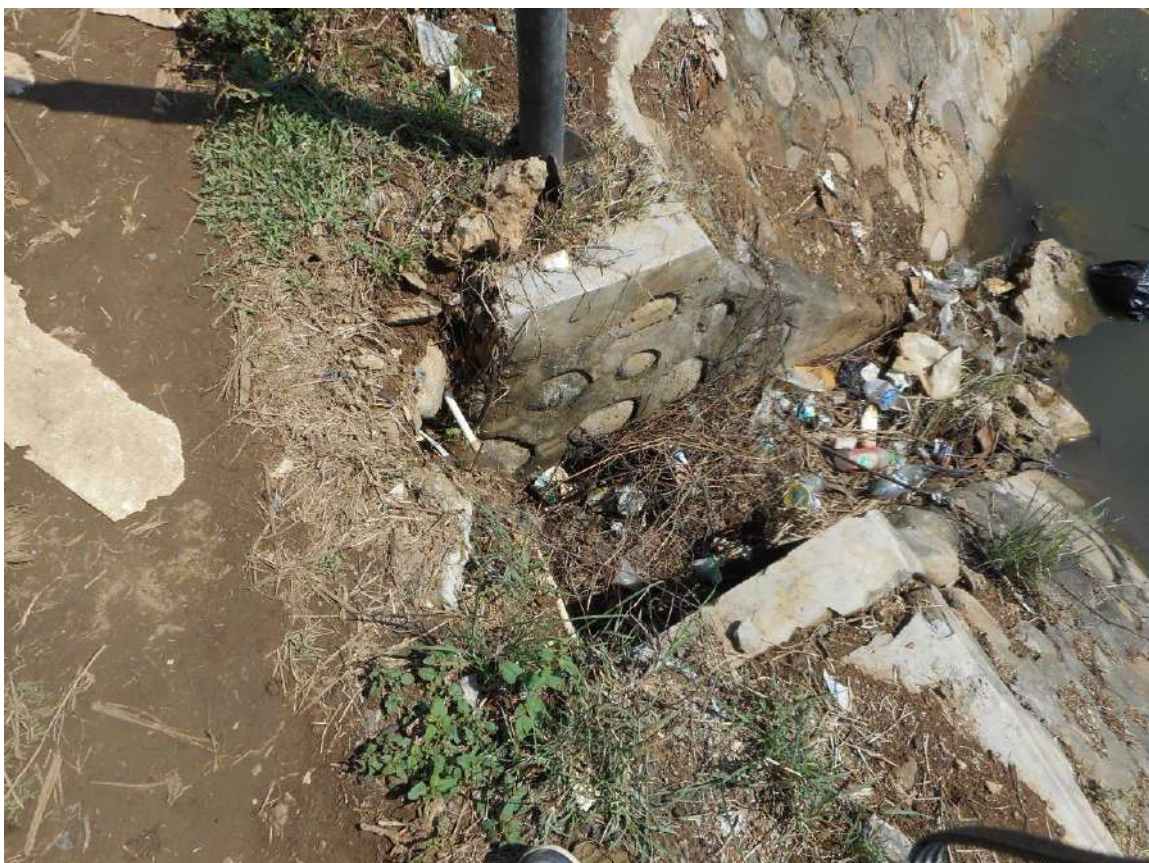
Photo 16 - Trash in drainage
