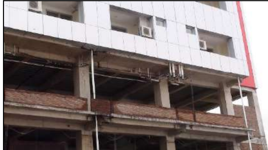
Figure 4.9: Building B,C,D; South side
