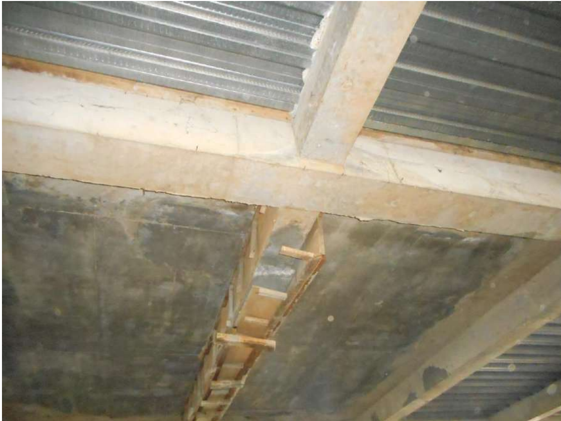
Photo 3 - Story 2 Beam Heavy Damage (Exposed)
