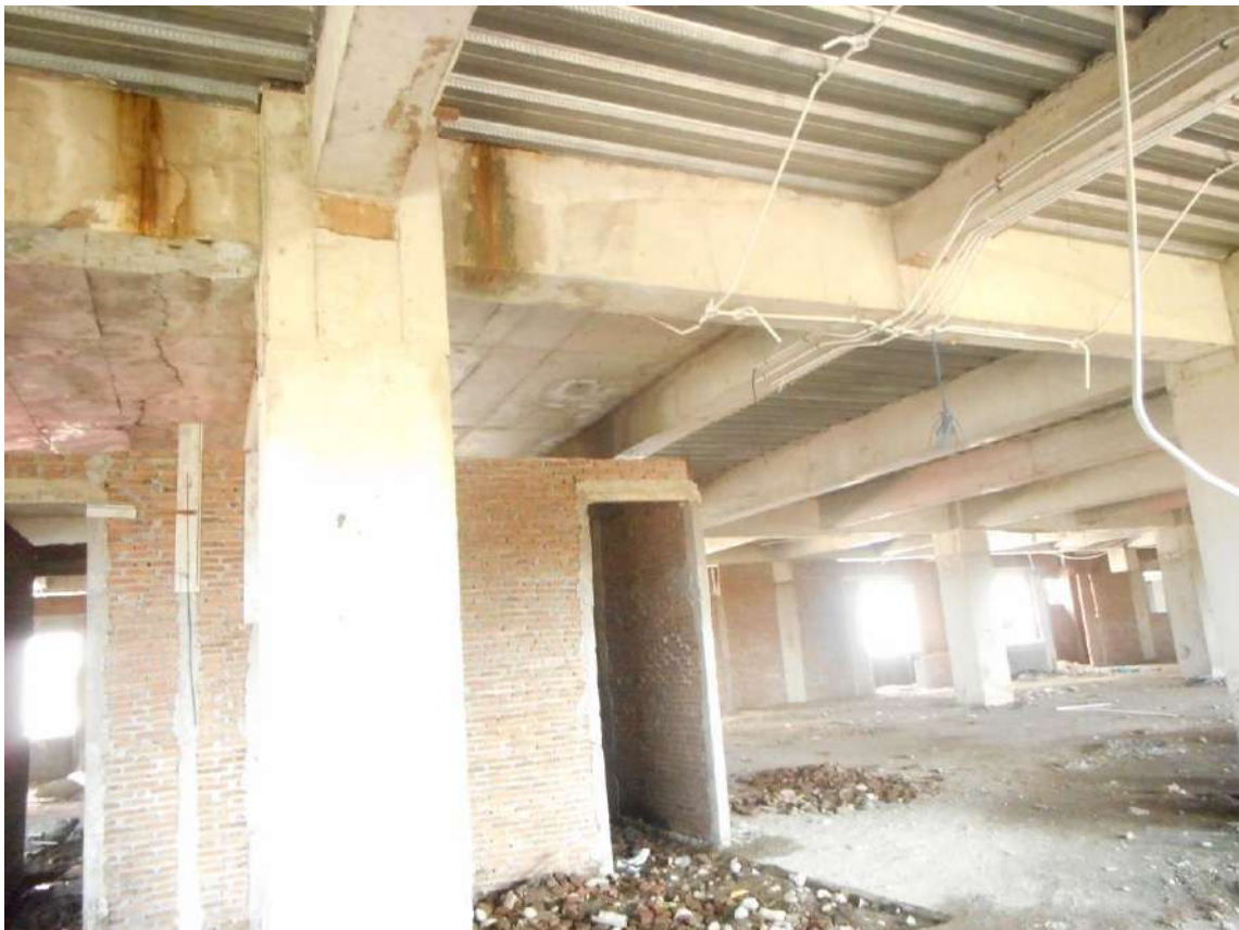
Photo 8 - Story 4 Corroded Reinforcement due to Leakage Water
