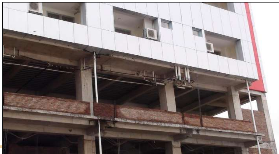
Figure 4.12: Unfinished Building B,C,D Exterior
