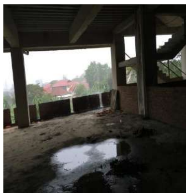
Figure 4.10: Unfinished area interior II
