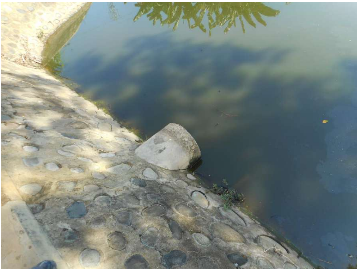
Photo 14 - Underground Pipe from Sump pit Basement to Pond
