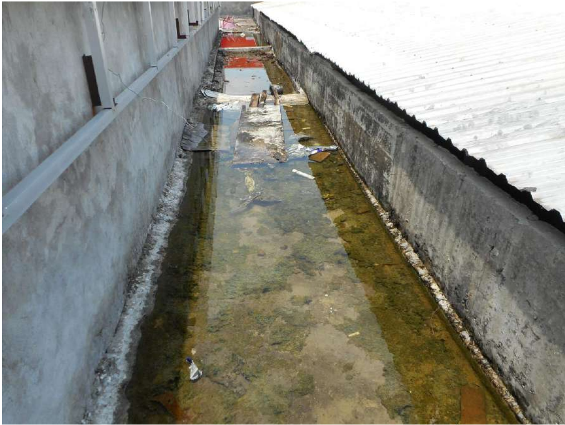
Photo 13 - Roof Drainage not Working
