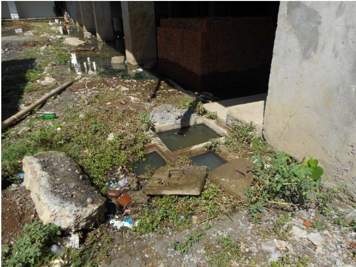
Photo 15 - Sump pit in Basement
